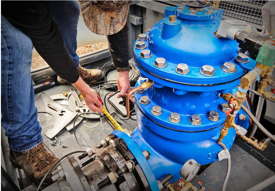
A miniature hydroelectric turbine that can generate electricity from water pipes
