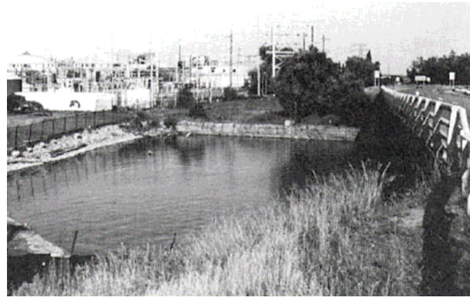
Photo of the area where the original Adams Plant Number One was erected (credit: T. Valone)
