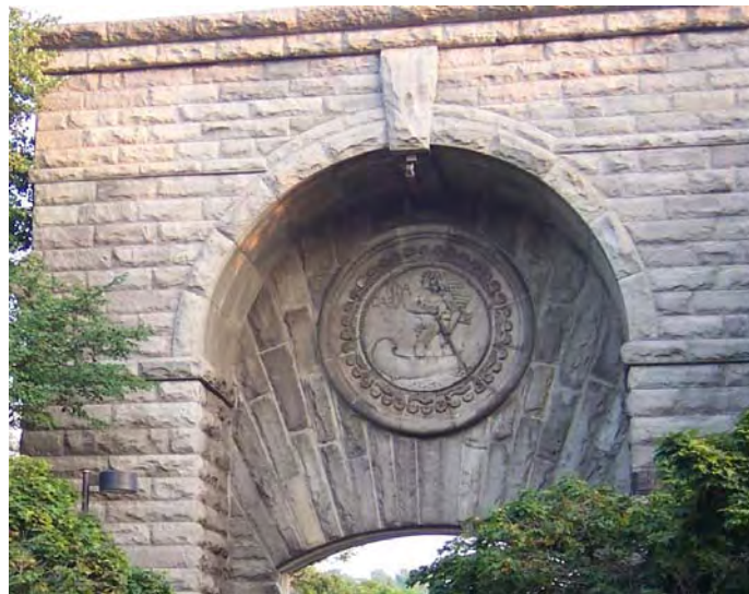
Adams Plant Number One Entrance Archway, the only remnant of this building that housed the original Tesla dynamos, is located behind Tesla's statue (credit: T. Valone)
