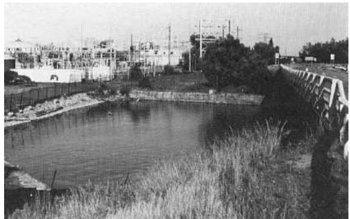
Photo of the area where the original Adams Plant Number One was erected
