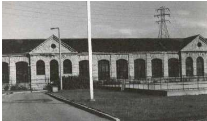
Adams Plant Number Three. The only original building out of the three still standing today.
